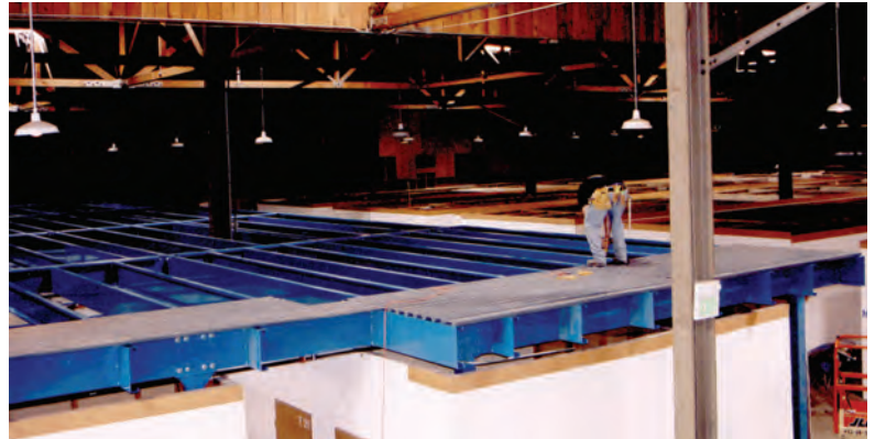
ResinDek® MD panels installed in 2003
